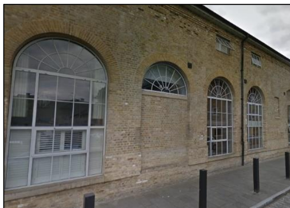
The former Goods Shed has been redeveloped
